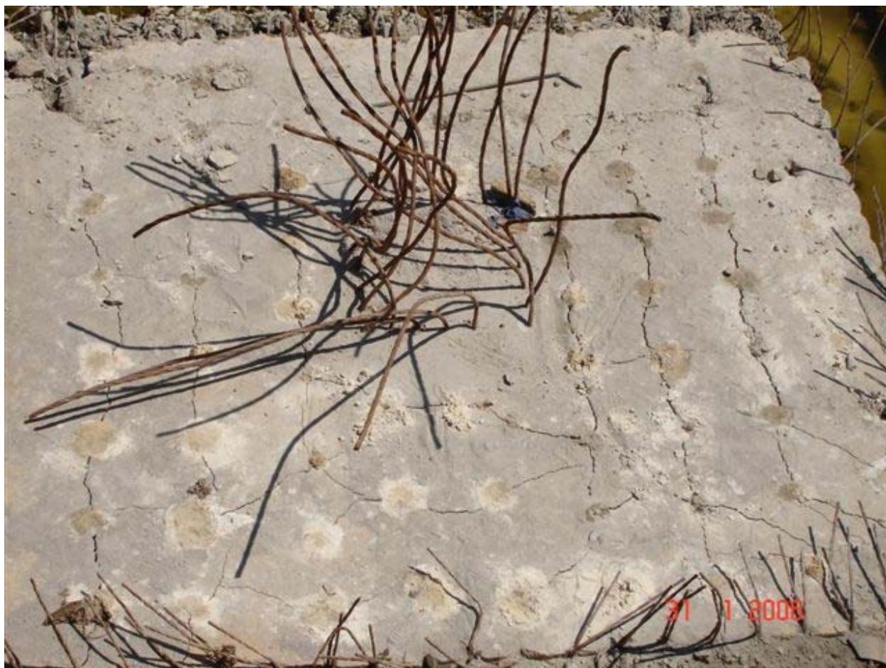
Reinforce concrete demoliton.
